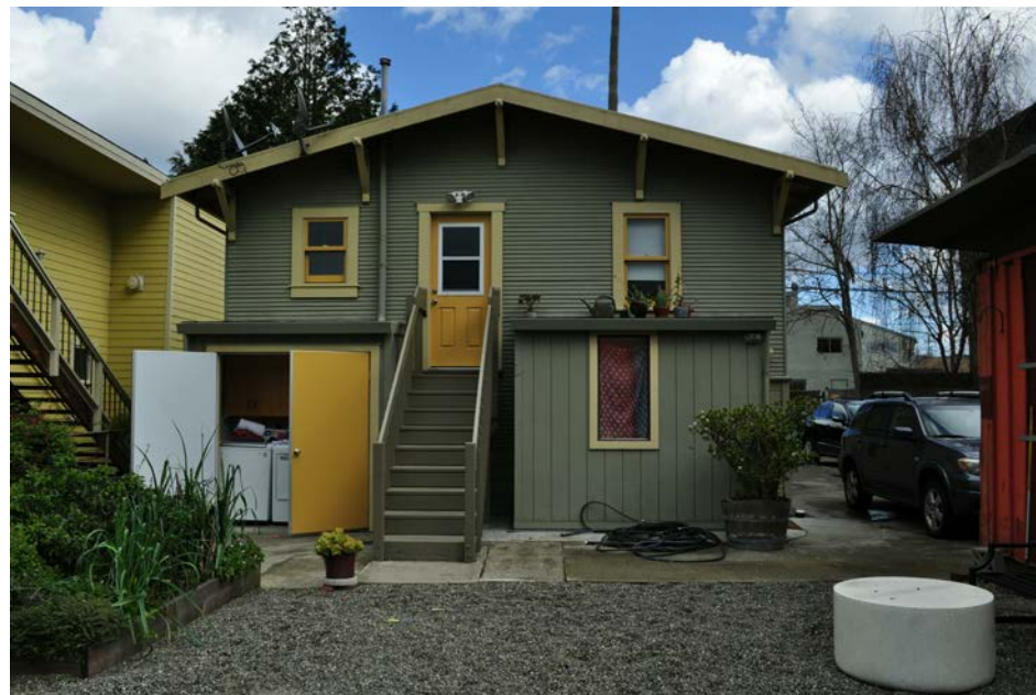
B - EXISTING BACK OF HOUSE
