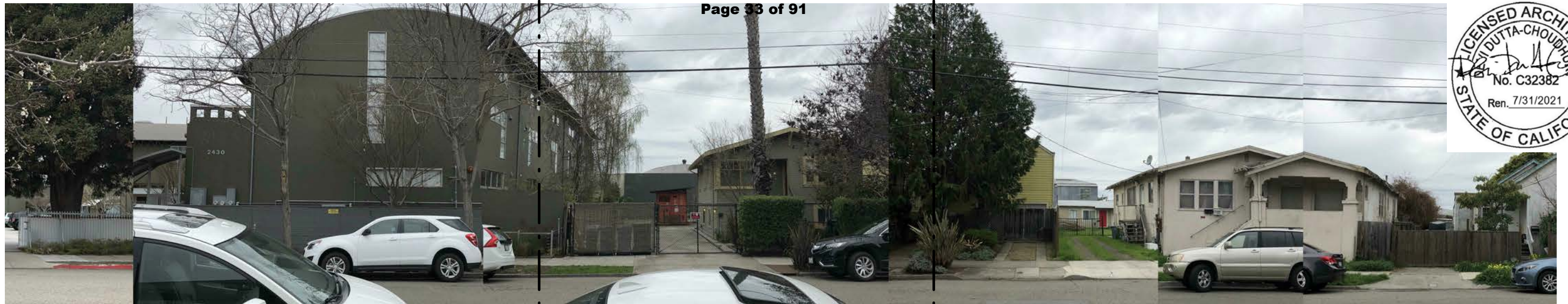
EXISTING WEST VIEW 2422 5TH STREET
